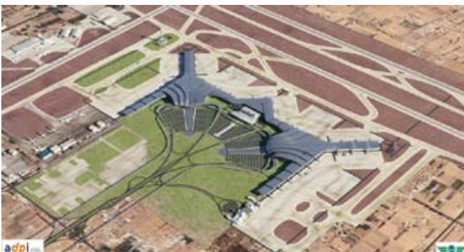
Tripoli International Airport – Aerial view of two new passenger terminals with existing terminal in the centre
